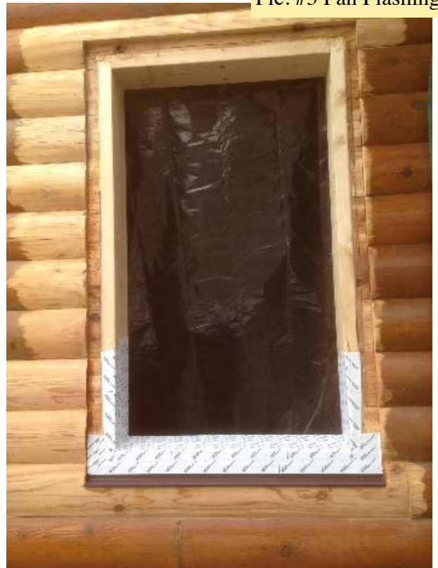
Pic. #3 Pan Flashing
